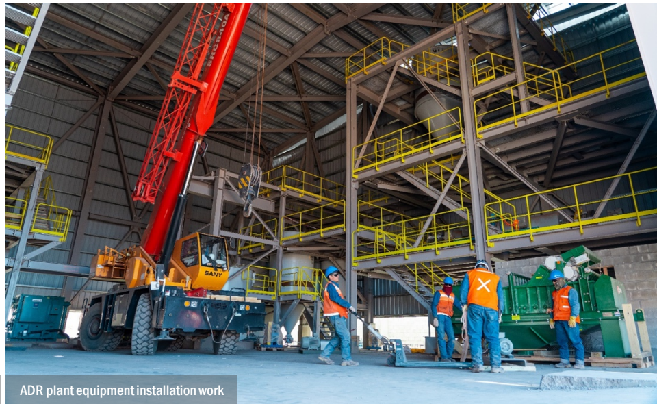
Panoramic view of ADR plant and refinery room
