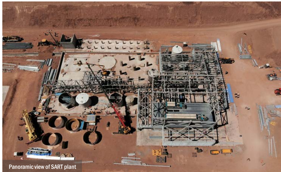
SART plant tank installation work
